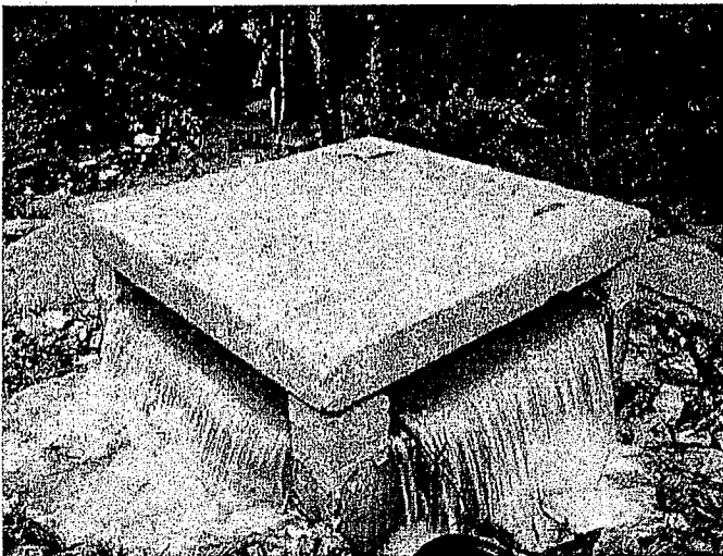
In Aberdeen, NC, a compact weir releases water on all sides, distributing stormwater to bioretention cells.
